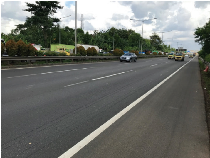
Figure 34: Trial section after 18 months of traffic
