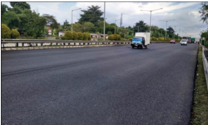
Figure 32: Visual on the 1st day of Open Traffic
