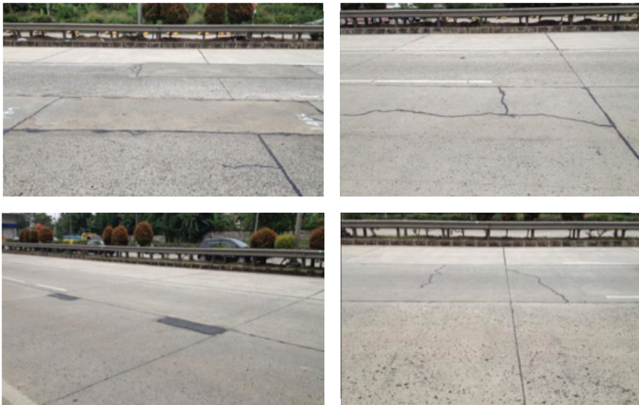
Figure 21: Joint and Crack Sealing on Existing Pavement
