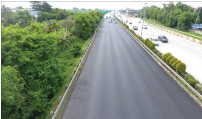
Figure 33: Visual on the 1st day of Open Traffic
