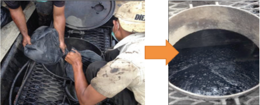
Figure 23: Binder preparation (adding RAR to the bitumen) at 175-185°C
