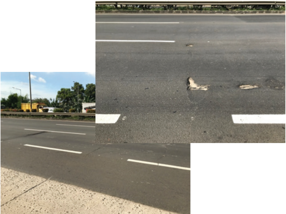
Figure 36: For comparison see Adjacent with the same pavement structure, same condition, and same traffic but with a Conventional Hotmix Section which is 2 months newer than the trial section and already has reflective cracks and many potholes
